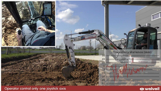
Example of mini-excavator activity with assisted function
